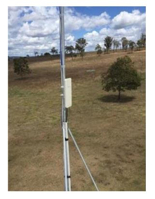
Point to Point connection antenna on a pole mount holding a Fixed Wireless antenna.
